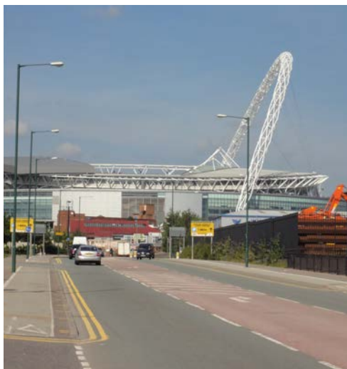
Picture 6.1 Great Central Way towards South Way - 'Stadium Access Corridor'
