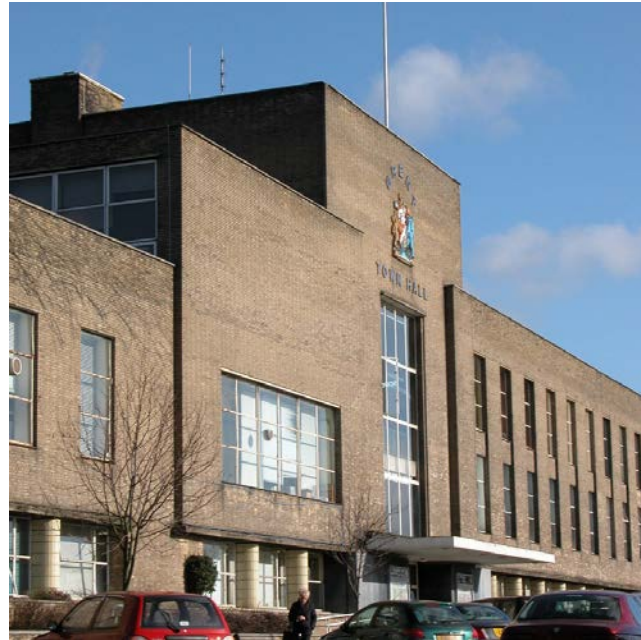
Picture 4.7 Brent Town Hall (Grade II)
