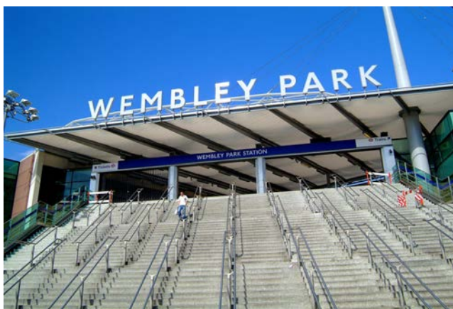
Picture 4.21 Wembley Park Station
