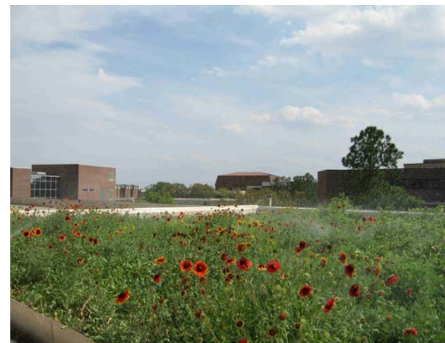
Picture 11.5 Example of a green roof
