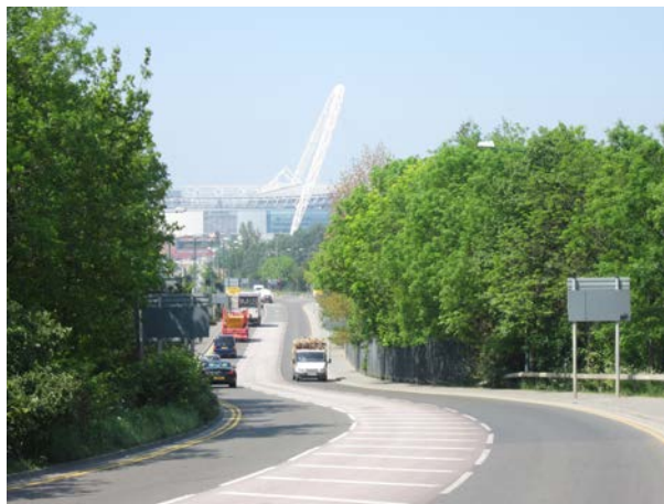
Picture 4.33 View of Wembley Stadium from the east
