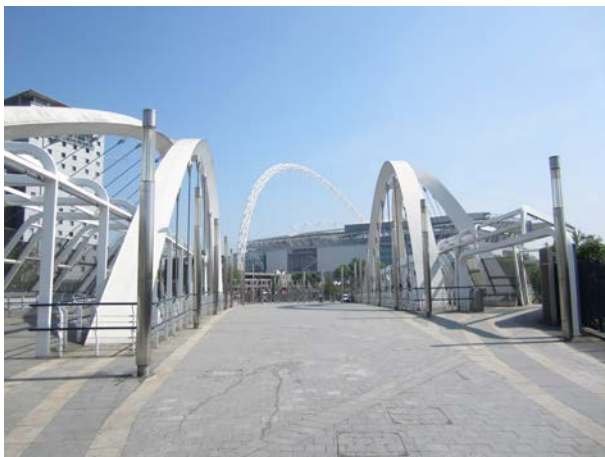
Picture 4.32 View of the Stadium from the White Horse Bridge
