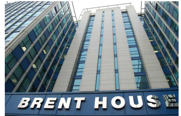
Picture 5.3 Brent House, Wembley High Road
