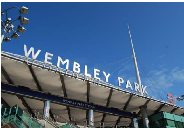
Picture 4.30 Wembley Park Station
